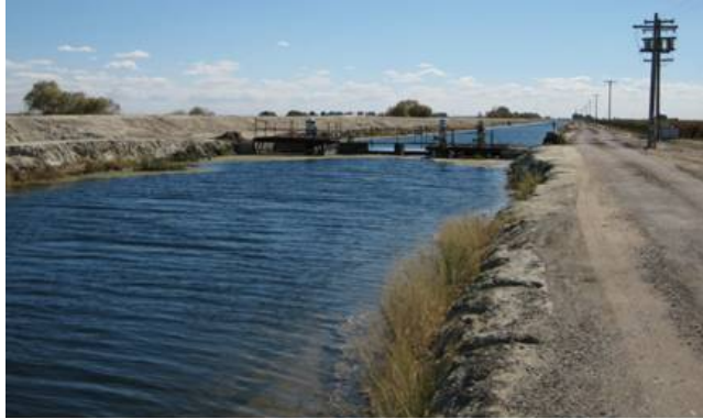
Figure 2. James ID Main Canal during pre-compaction seepage test.
