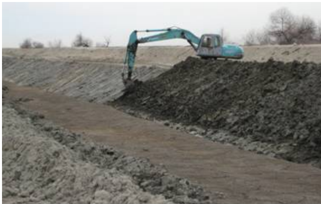
Figure 3. James ID Main Canal during side compaction
