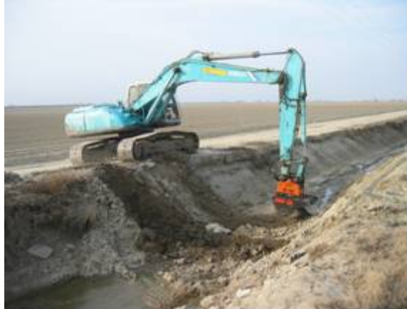
Figure 6. Compacting the sides and bottom of Lateral H at James ID
